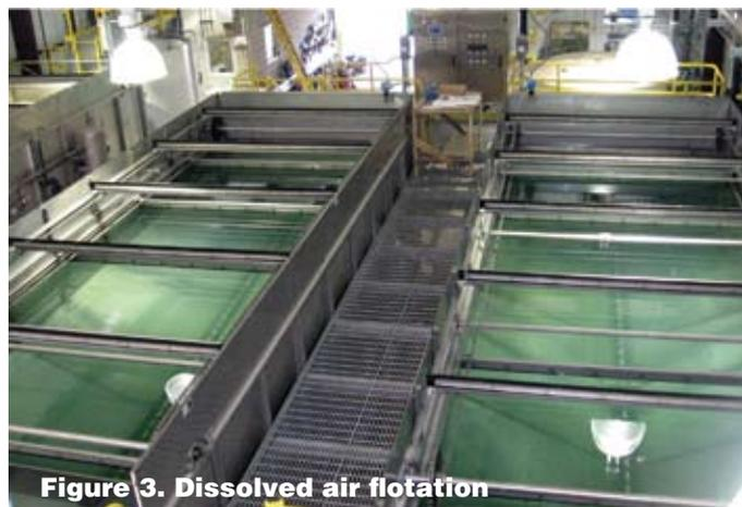
**Figure 3. Dissolved air flotation**
